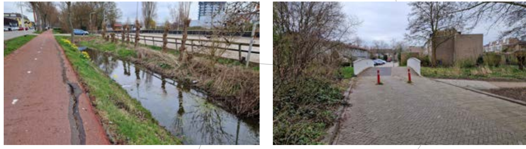
Bike path with sloped verge. Cycling poles without light or rib marking, preventing cars from crossing the bridge. Delft, Ruben van de Boel.
